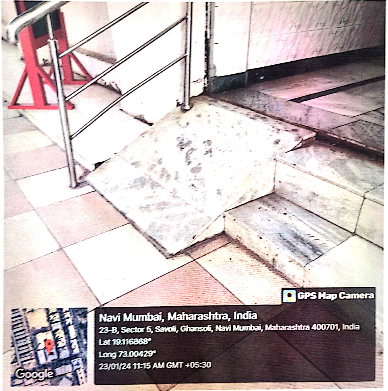
Geotagged Photo of Ramp
